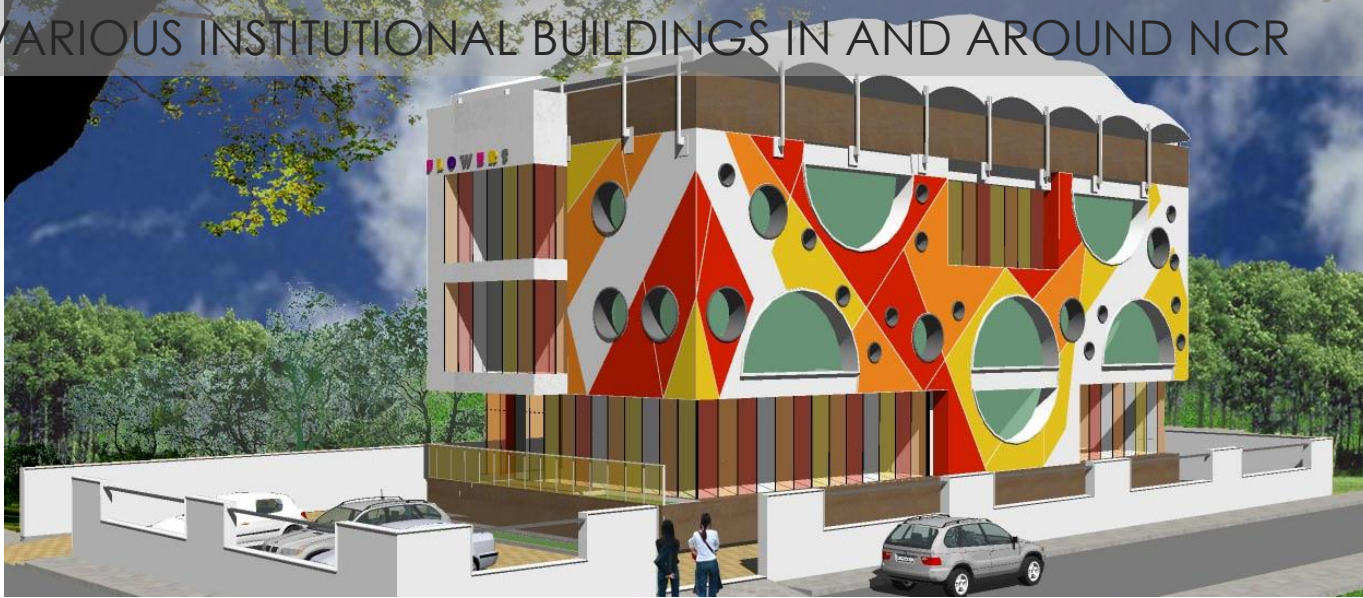
PRIMARY SCHOOL, LOCATION: FARIDABAD CLIENT: ST. JOHN'S SCHOOL SOCIETY STATUS: ONGOING
